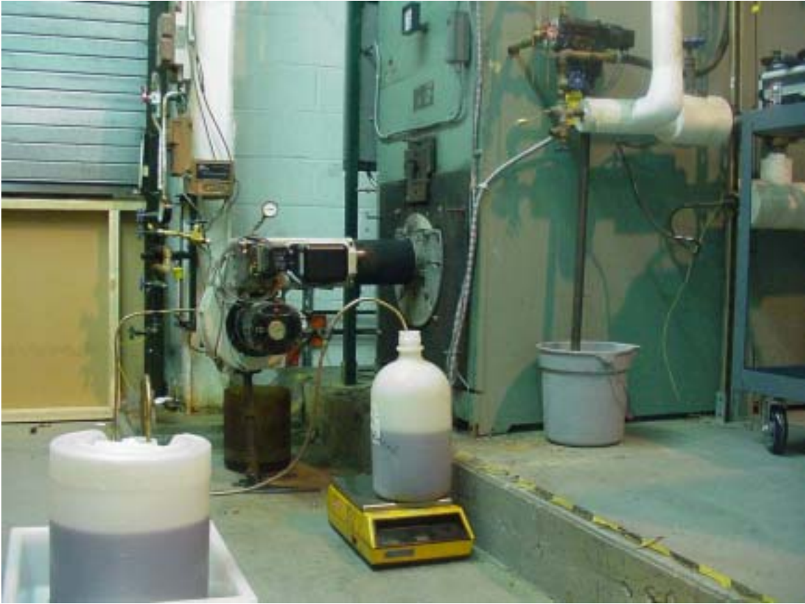
Figure 2. Commercial Boiler Set Up
