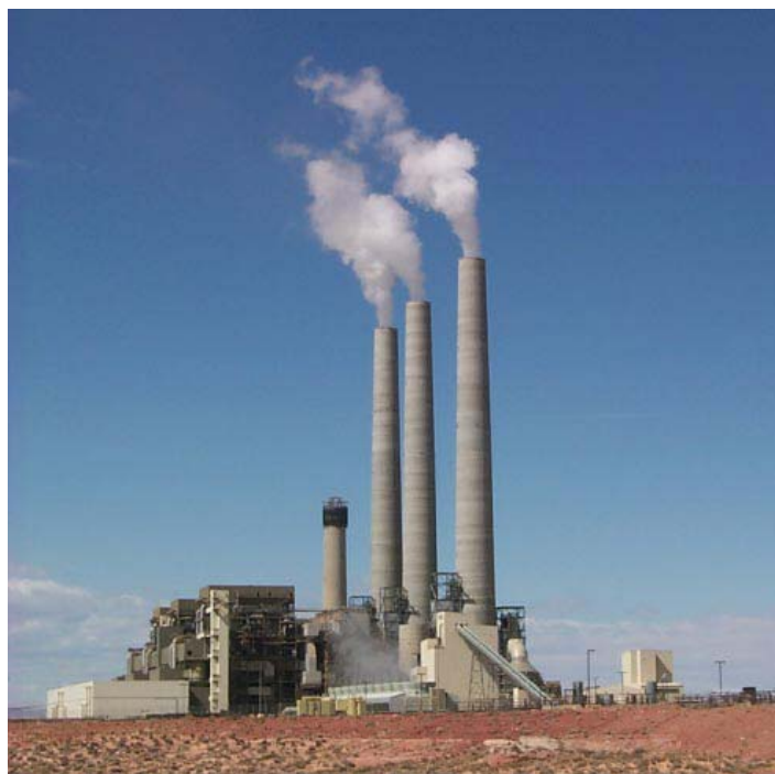
Navajo Power Plant
