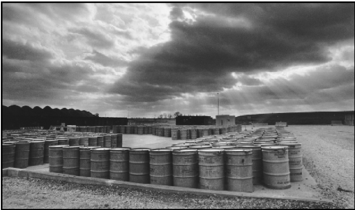
Barrels of transuranic waste sit on a concrete pad in temporary storage. This waste is contaminated with traces of plutonium. More than 300,000 barrels of such waste from nuclear weapons production are buried or stored around the country. Cleanup efforts throughout the weapons complex will add to the volume of this waste. Transuranic Waste Storage Pads, E Area Burial Grounds, Savannah River Site, South Carolina. January 7, 1994.
