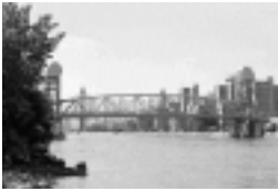
FIGURE 1 The Roosevelt Island Bridge over the East River in New York City is an example of a vertical lift bridge. (Courtesy of Mead & Hunt, Inc.)
