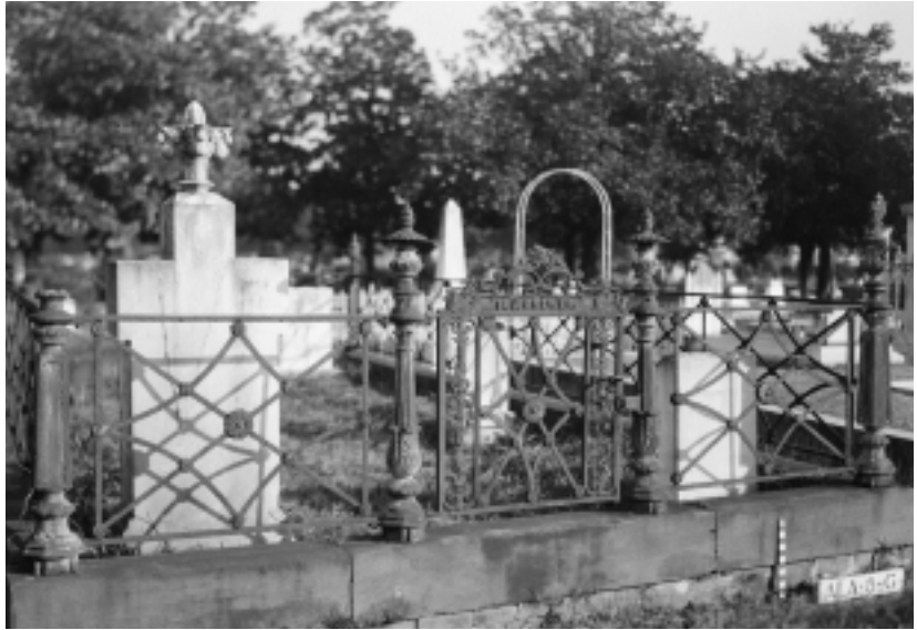
FIGURE 6 HABS documented the cast iron fence at Magnolia Cemetery in Mobile, AL. Note the serial number and scale in the lower right-hand corner. (E.W. Russell, photographer, February 1963. Courtesy of the Library of Congress, Prints and Photographs Division.)
