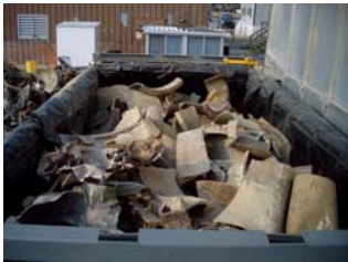
Steel Plate loaded too high in container.
