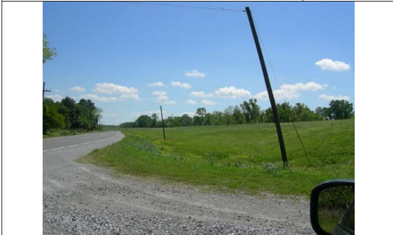
Photo 20: View along Mississippi River levee south of site, facing south.
