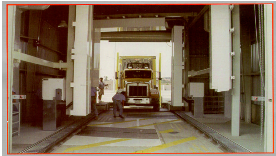
Figure 2: Typical Fixed-Site Truck X-Ray
