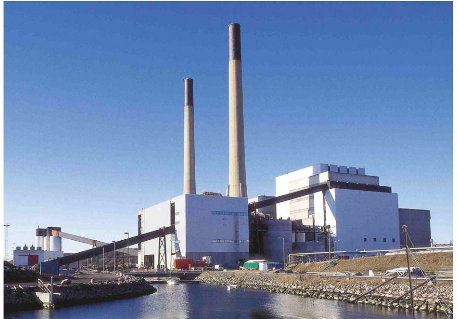
CT-121 FGD Plant at Stignæs Power Station, Denmark
