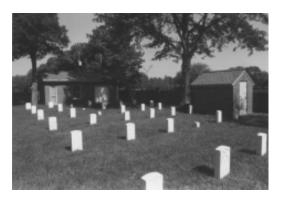
A brick and concrete pump house, 11 feet by 7 feet, was constructed in 1927. A brick and concrete utility building with comfort station, 26 feet, 6 inches by 11 feet, 6 inches, was constructed in 1933. The roof is clad with asphalt shingles. A brick and concrete gasoline storage building, eight feet five inches by eight feet, was constructed in 1936. Its roof is clad with asphalt shingles.
