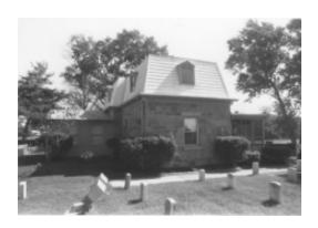
story are six-over-six double hung, while the upper-story windows are casement types with two panes in each casement. The interior retains much of the original fabric. It is finished with hardwood floors and plastered walls and ceilings. A brick and frame kitchen lean-to addition on the rear was constructed in the early 1900s. In 1925, a concrete front porch floor replaced the wood floor. A buff-colored brick garage with stone inserts was added in the 1950s.
