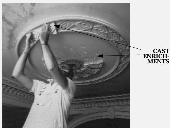
Fig. B. Ornament layout is determined using plane geometric principles; segmented locations are deeply scratched to provide a rough surface for adequate bonding using plaster as an adhesive. Photo by Peter Sanders.
