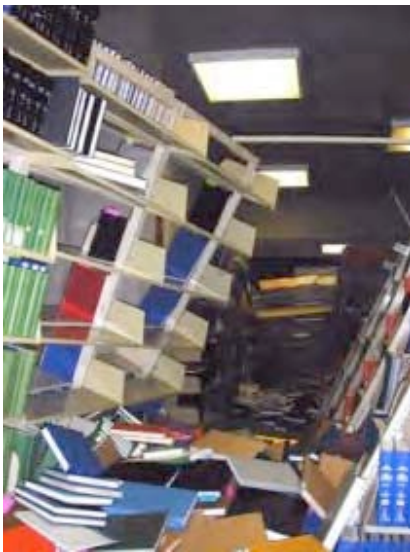
A rolling 6.8 earthquake on February 28, 2001 knocked tens of thousands of books off the shelves, damaged stack ranges, and affected library services at the University of Washington in Seattle.
