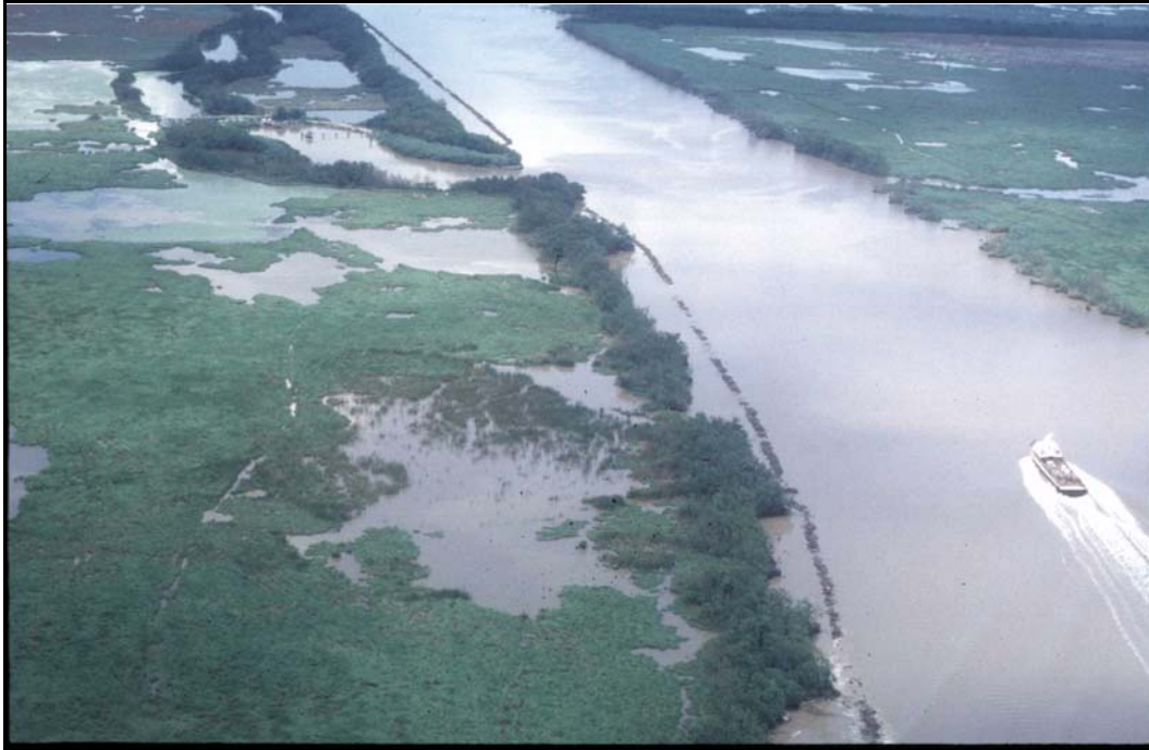
Figure 2. Photo of the Freshwater Bayou Canal channel between CTU 1 (left side) and reference area R2 (right side) showing part of the ME-04 rock dike, deteriorated spoil banks, and ponded areas in the marsh along both sides of the channel.
