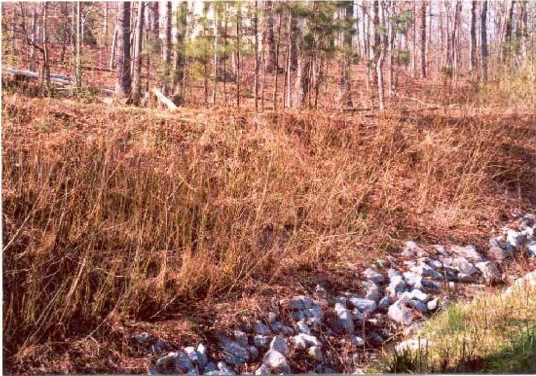
Urban Streambank Stabilization – Gwinnett County
