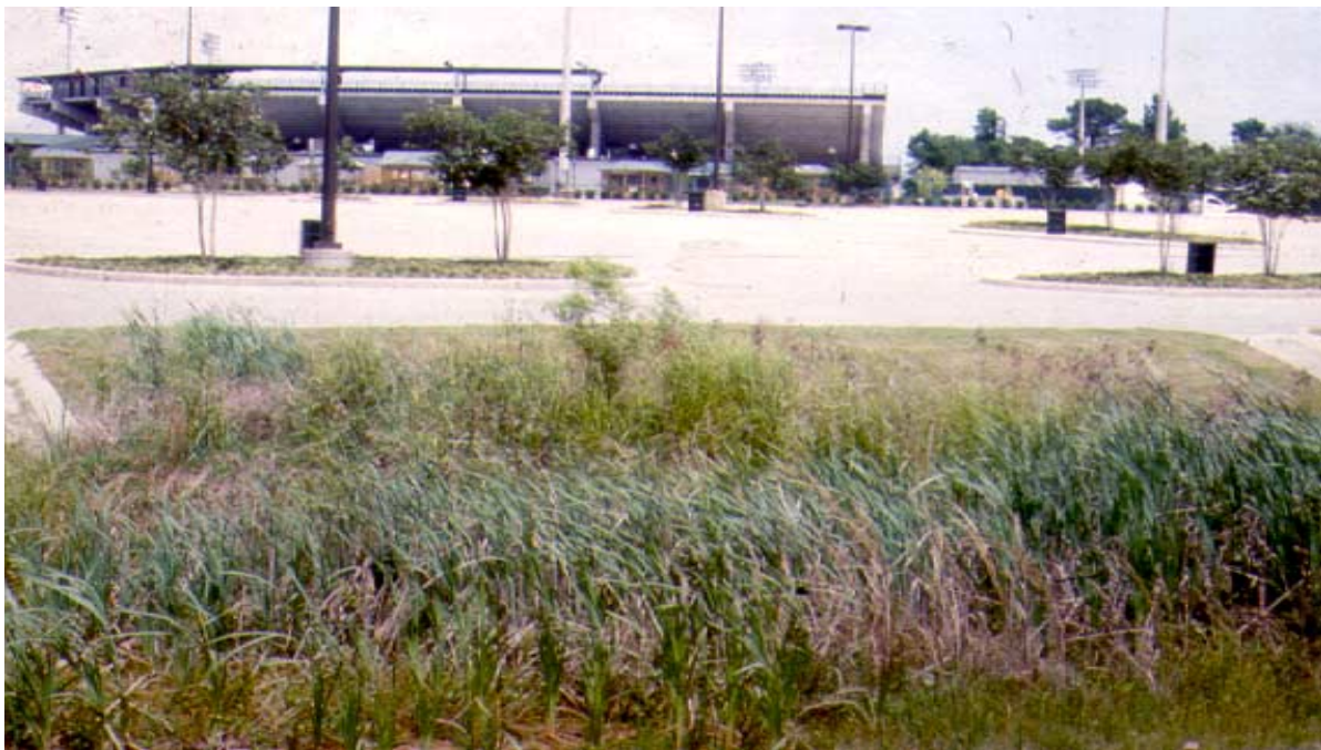
Mobile, AL – Stormwater Constructed Wetland treats runoff from parking lot at Hank Aaron Baseball Stadium.
