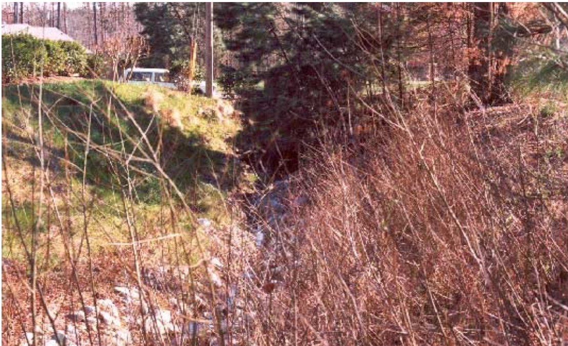
Urban Streambank Stabilization – Gwinnett County
