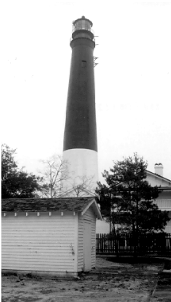
Figure 4. Brick masonry construction in the 171-foot-tall Pensacola Lighthouse in Florida.
