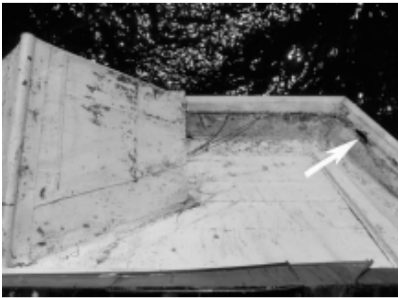
Figure 18. View of built-in gutter on a caisson lighthouse; arrow indicates fist-size hole. This condition must be treated before mothballing.
