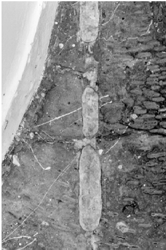
Figure 32. This sheet-copper-covered lantern gallery deck has been repaired several times by soldering sheet copper patches over the holes. This method of repair, if performed properly, greatly increases the life span of the roof covering.
