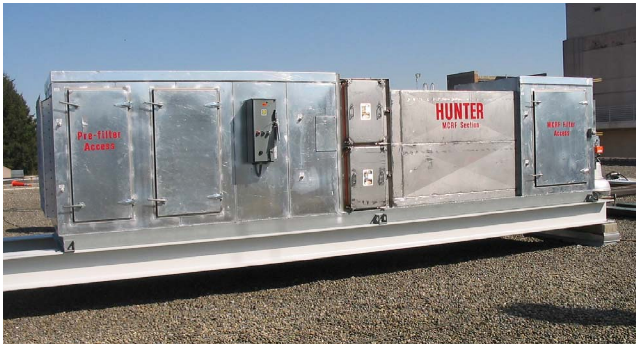
Figure G-12. Multi-Cell Radial-Flow (MCRF) Filtration Unit
