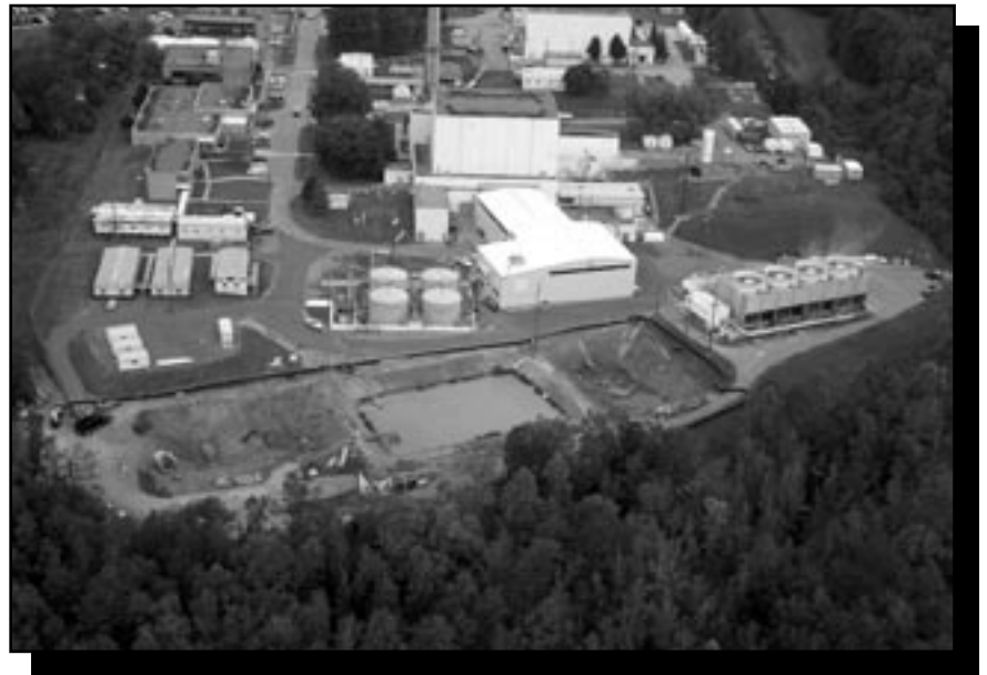
HFIR impoundments during excavation
