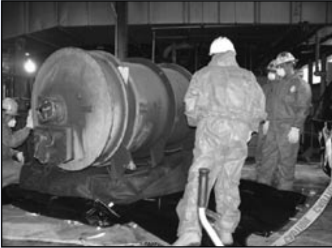
Converter removal and shipment from the K-25 Building
