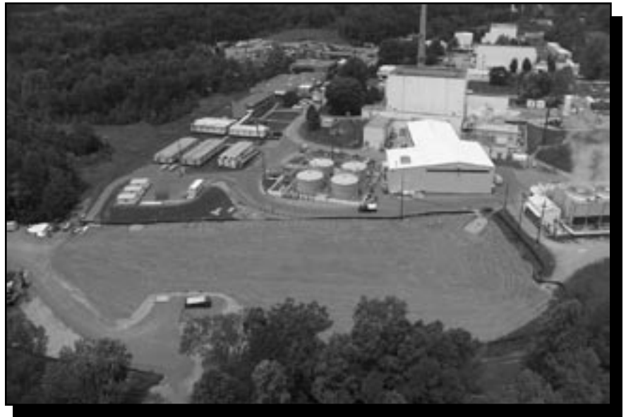
HFIR Impoundments after excavation
