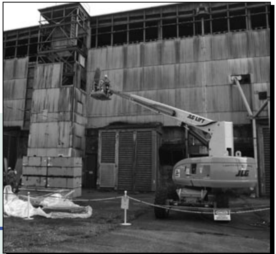
Transite removal from the K-25 Building
