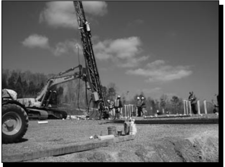
Workers are driving sleeve pipes at Trench 7
