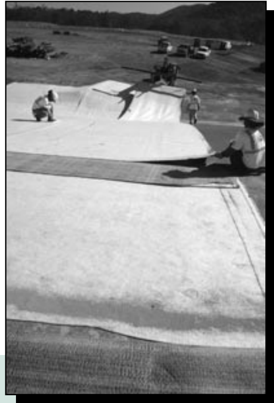
Liner being placed at SWSA 5 (above), and SWSA 6 (below) after remediation (June 2006)
