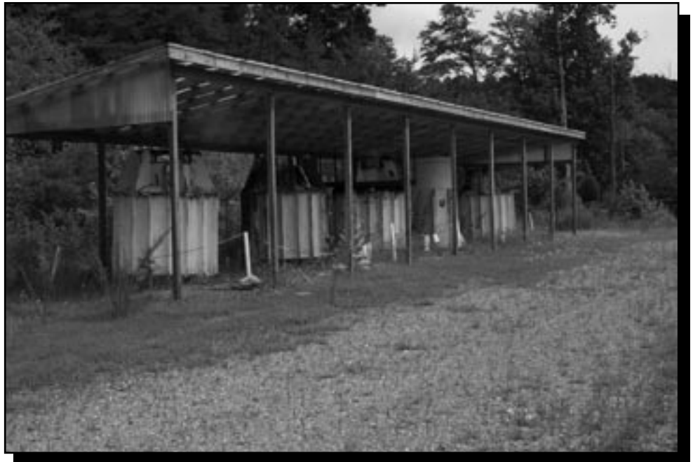
Shielded transfer tanks
