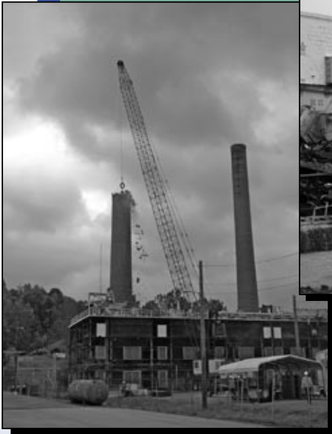
K-1501 stack demolition
