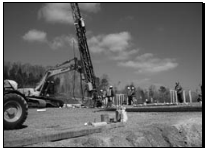
Trench 7 at Melton Valley
