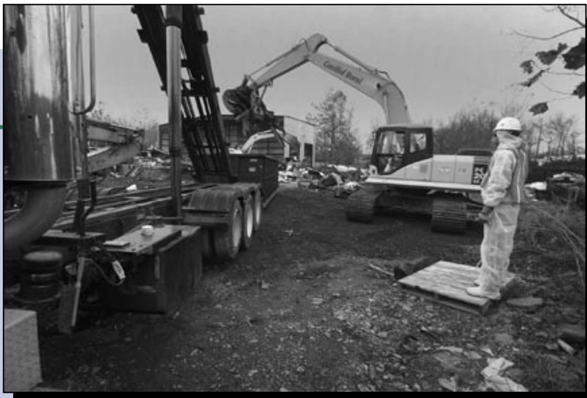
Debris removal at the DWI 901 Site
