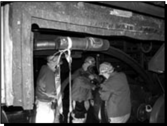
Foam injection into K-25 piping to stabilize the contents
