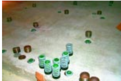
Figure 5. Vibration isolator elements and leveling devices being installed.
