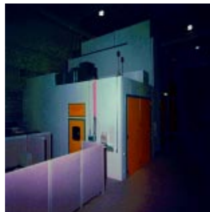
Figure 2. Finished chamber complex within high-bay test facility with crane and floor access services.
