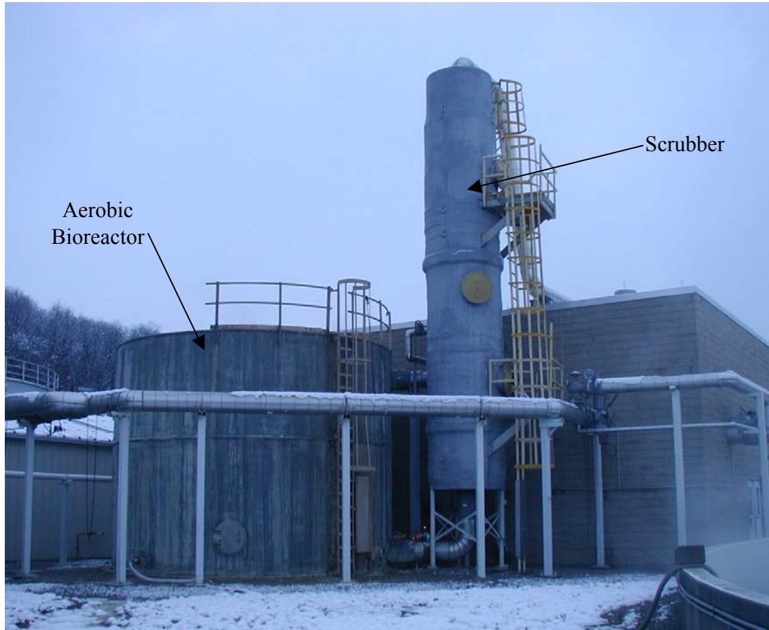
Figure 1-2. THIOPAQ System Tested
