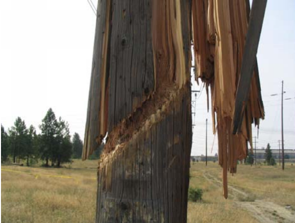
13.8 Kv Kaiser Feeder power line west pole showing red M/R blade strike when aircraft was inverted.
