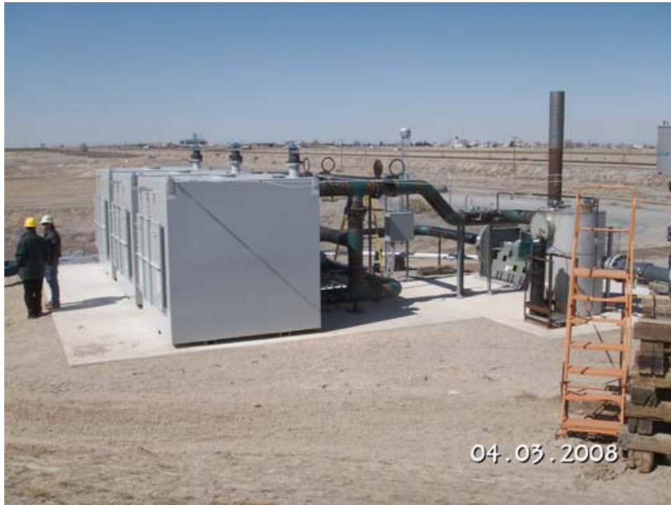
FMC Pond 16S. The large square vessels are the carbon filters that treat the gas to safe levels before discharging to the air. EPA photo
