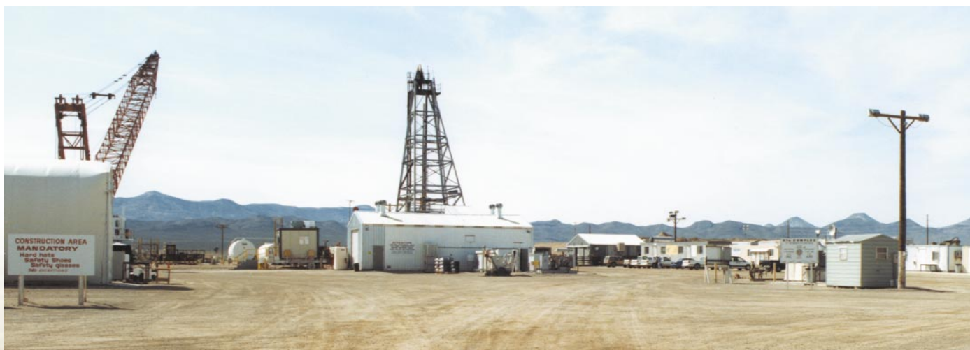
The U1A complex at the Nevada Test Site consists of several buildings and instrumentation trailers from which scientists monitor experiments conducted underground.
