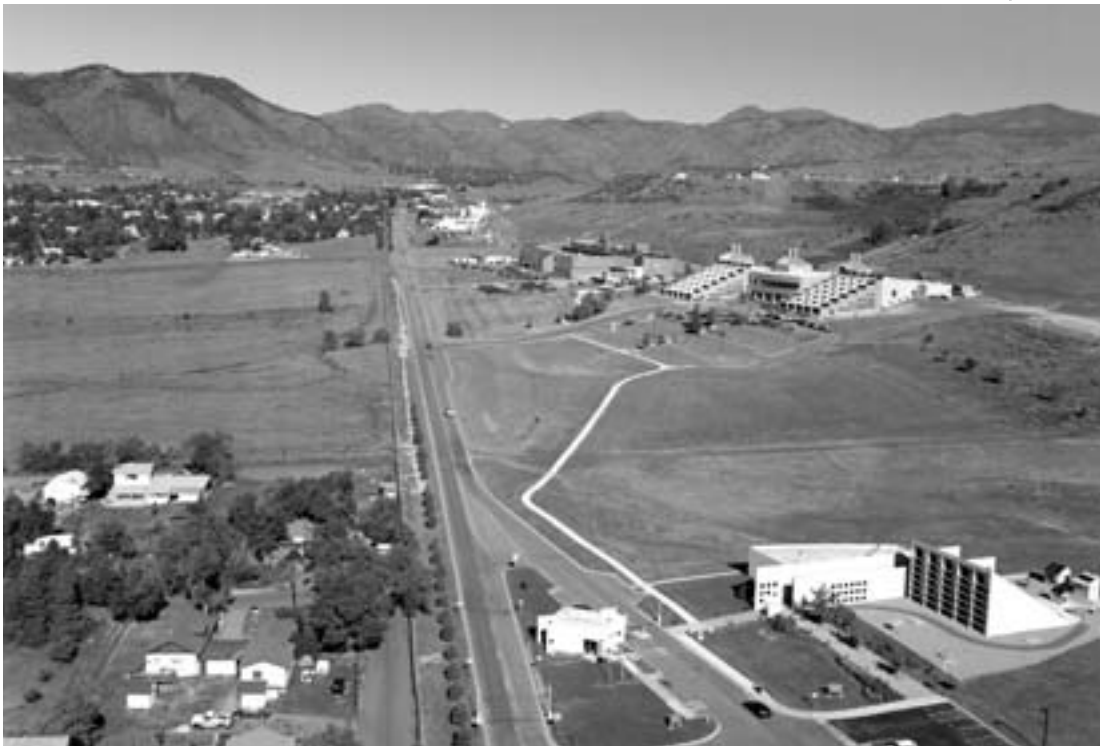
This aerial photo shows NREL's primary research facilities at the South Table Mountain site. In cooperation with the state and county, the mountain's mesa sides and top were put into open space easement in exchange for 25 acres of additional buildable land adjacent to the primary research site.
