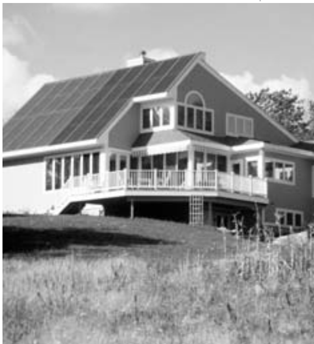
This house in coastal Maine generates its own electricity from a 4.25 kW PV system. Through a net-metering relationship with Central Maine Power, surplus solar electricity is exported to the utility grid, effectively spinning the utility meter backward. The owners get this power back in an even exchange at night, and during periods of low sun.
