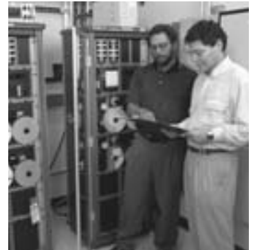
Located at the Solar Energy Research Facility, these control panels monitor the potential release of toxic gases.
