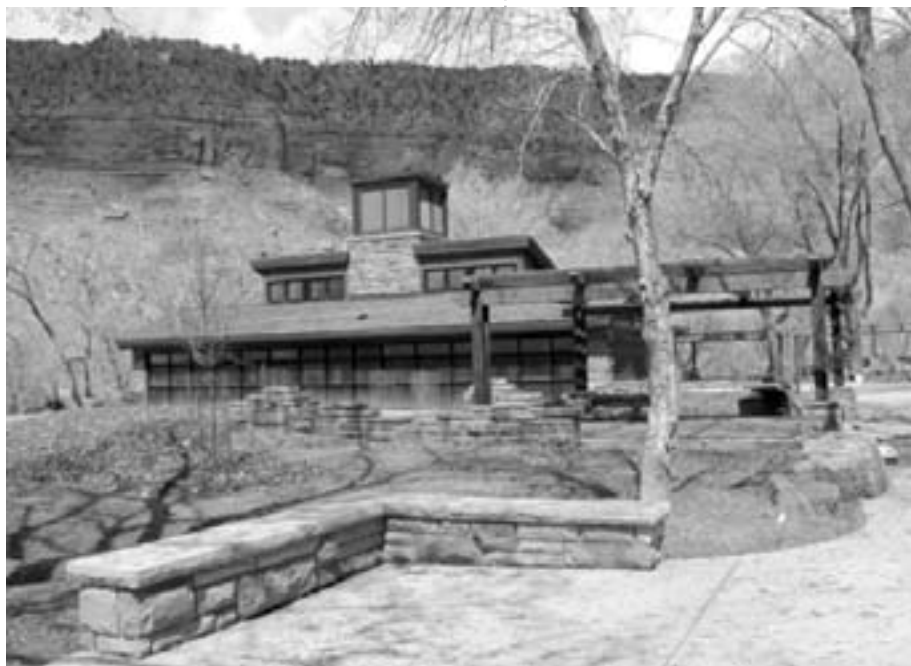
The National Park Service and NREL worked together to create this energy-efficient complex, the 7,600-square-foot Zion National Park Visitor Center. The building includes a 1,100-square-foot comfort station featuring daylighting, Trombe walls for passive solar heating, downdraft cooltowers for natural ventilation cooling, energy efficient lighting, and advanced building controls. These features are expected to result in energy cost savings of about $16,000 per year.
