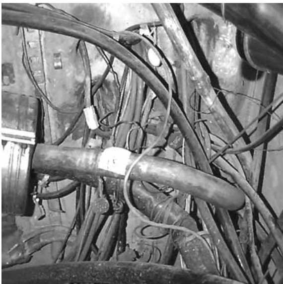
OLD WIRES were replaced in the ECIM project.
