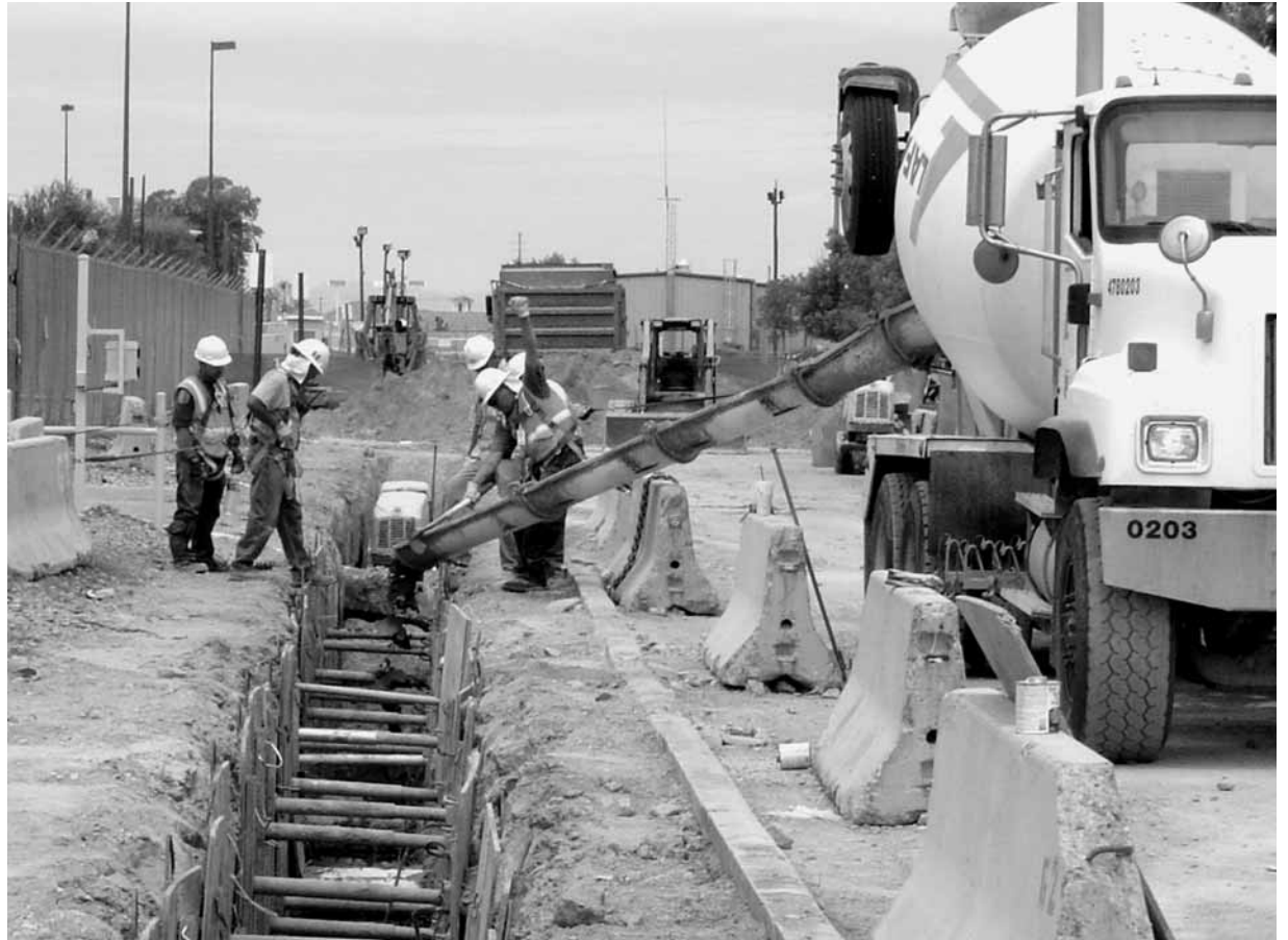
ECIM CONSTRUCTION WORK took 31 months to complete. The underground work involved tearing up streets, sidewalks, landscaped areas, and parking lots and trenching as deep as 16 feet so that duct banks could be installed. (Photo by David Hendrix)
