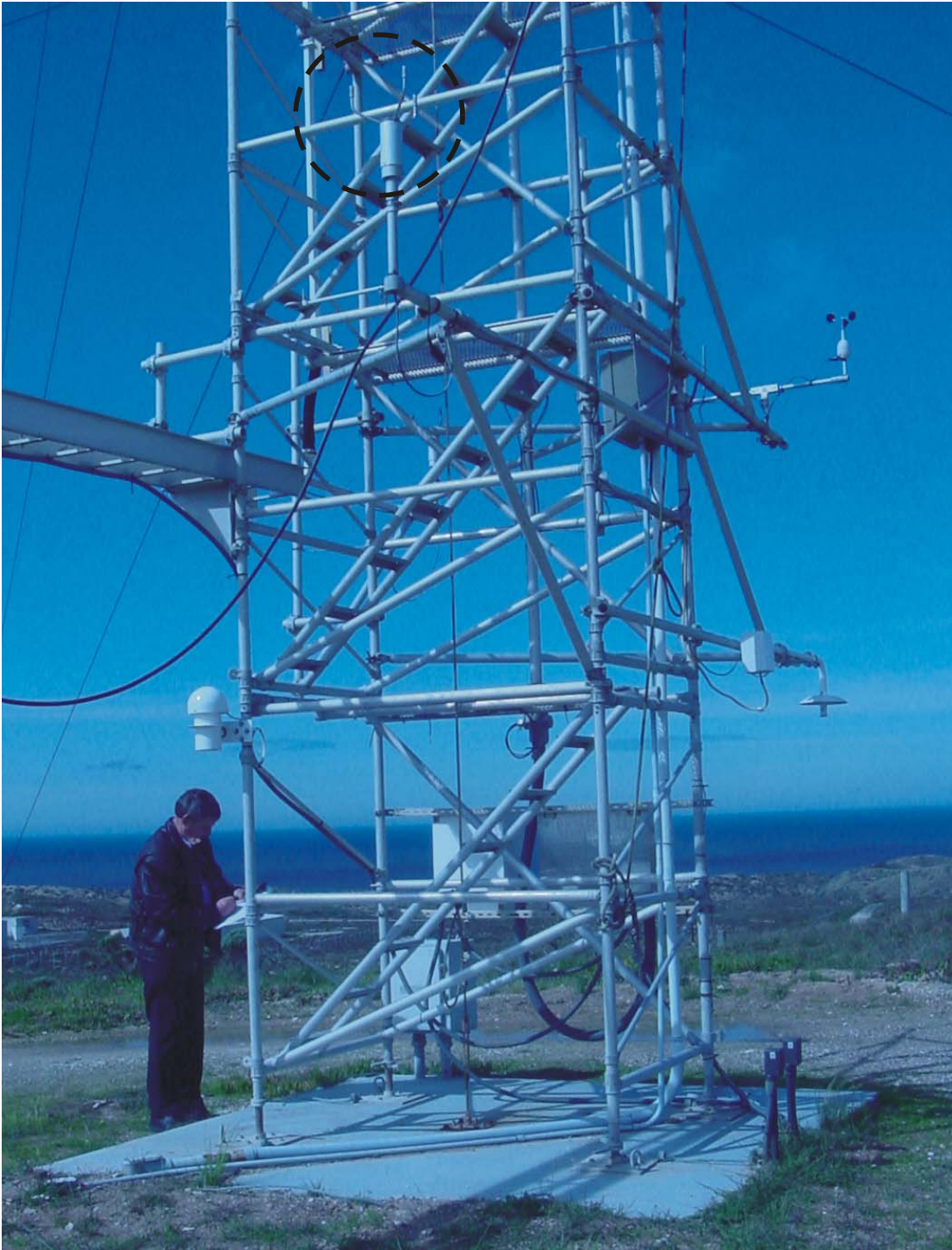
Figure 1. Legacy and RSA wind sensors at the 12 ft level on Tower 102 at the WR. The Legacy cups can be seen in the middle-right. The Legacy wind vane is obscured by the electronics box. The RSA1 ultrasonic sensors can be seen in upper-center, inside the dashed black circle.
