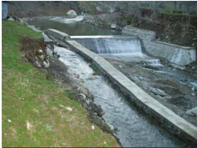
Fig. 5: PRB water diversion dam ready for final inspection
