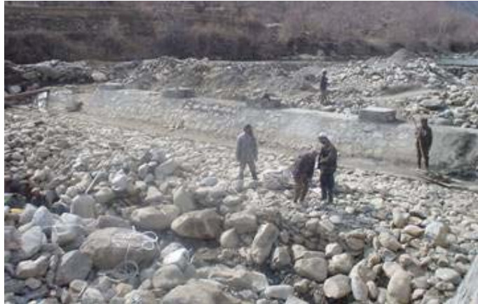
Fig. 14: Mahigeer water diversion dam, construction advance
