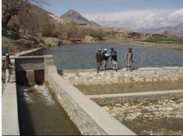
Fig. 4: Final Inspection of HAFO water diversion dam
