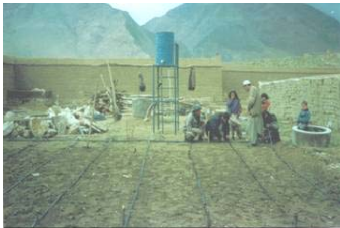
Fig. 8: Drip Irrigation Installation
