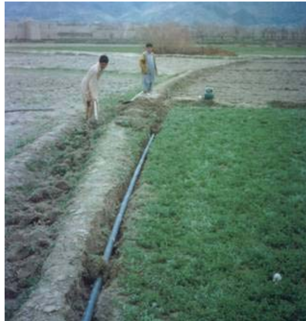
Fig. 15: Installation of main water line for drip irrigation commercial garden
