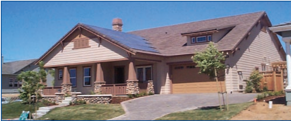
Southwest view of the Centex 21st Century Performance Home in Livermore shows 3.6-kW photovoltaic panels on the south-facing roof.
