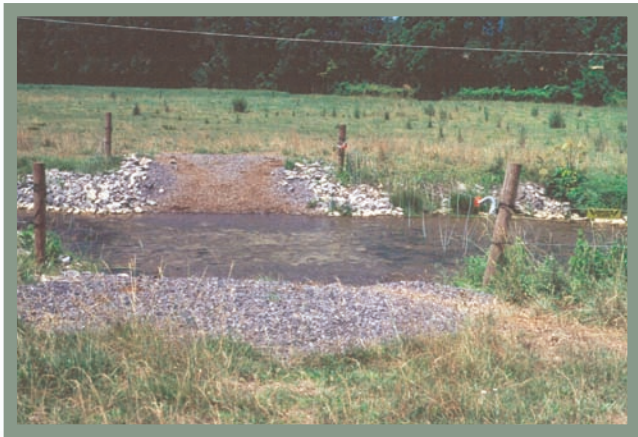
Figure 5. Crossings were installed to allow livestock limited access to the stream.
