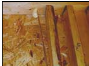
Penetration is sealed with foam caulk.
