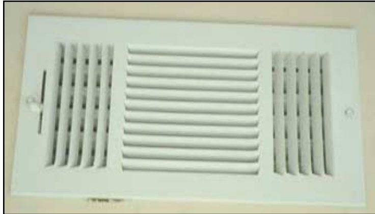
Gaps in the drywall can be air leakage sites.
