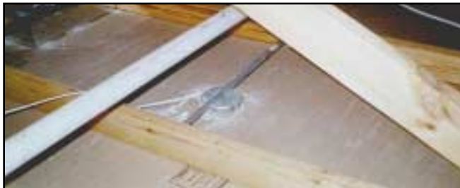
Before the ceiling is insulated, caulk around all holes that were made through the sheetrock.
