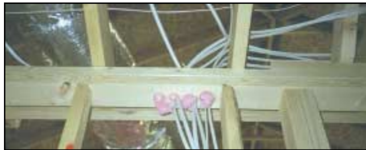
Foam all penetrations in the top plates.
