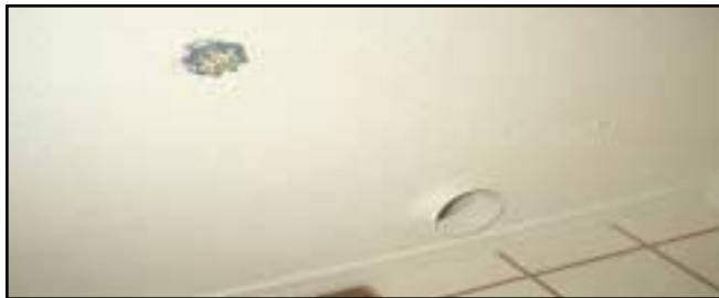
This is an excellent example of a finished dryer vent and water shut-off valve.
