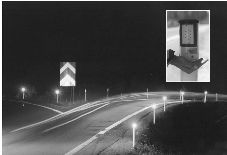
Fig. 4. Light-emitting diode lighting (LEDs). Emerging applications for LEDs promise significant energy savings. They are already widely used in red and green roadway signal lighting and Exit signs. Transportation officials cite safety benefits due to improved visibility and reliability (far longer service life and lower maintenance costs than traditional lamps) (Said, 2001; Prey, 2001). Moreover, they can be economically powered by photovoltaics with backup batteries, to ensure availability during periods of power outages. White LEDs are also beginning to be used for way-lighting, promising significantly reduced energy use and improved safety (Borg, 2001). The photo shows tests underway on Swedish roadway (Orreberget) known for high accident rates. Each pole requires only 3 W of power, which corresponds to lighting energy demand reduction of up to 90% compared to standard lighting systems. In preliminary evaluations drivers have reacted positively. Tests currently underway or planned in Sweden cover 17 miles of roadway, and approximately 800 poles. The inset shows an individual pole head using 10 LEDs (current systems require only 4 LEDs).
