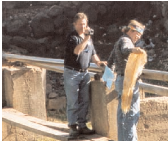
GRAY LOWREY (6216, left) videotapes a leaking pipe during his Rotary International Group Scientific Exchange in Mexico.
