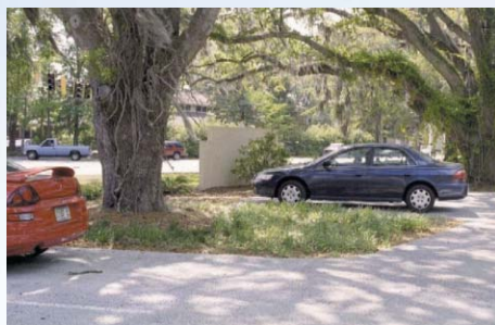
High-albedo pervious pavement supports light traffic while mitigating the heat island effect and allowing stormwater to pass through.
