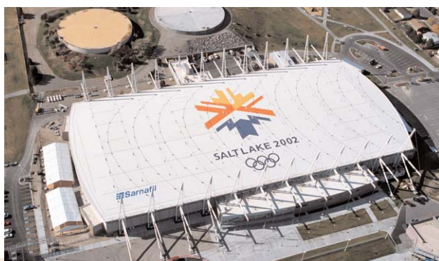
The Utah Olympic Oval used cool roof technology.
