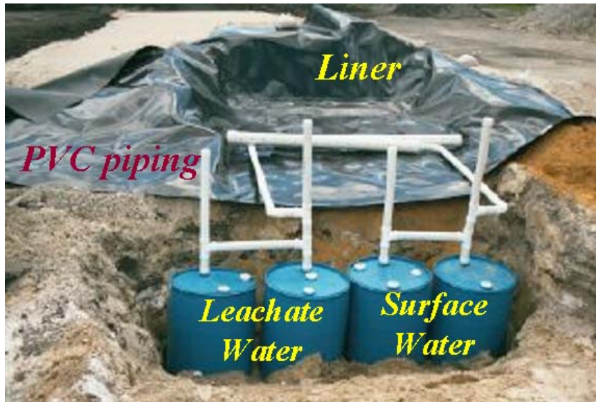
Figure 3.11 Photograph of Limerock Collection Systems prior to backfilling with Limerock
