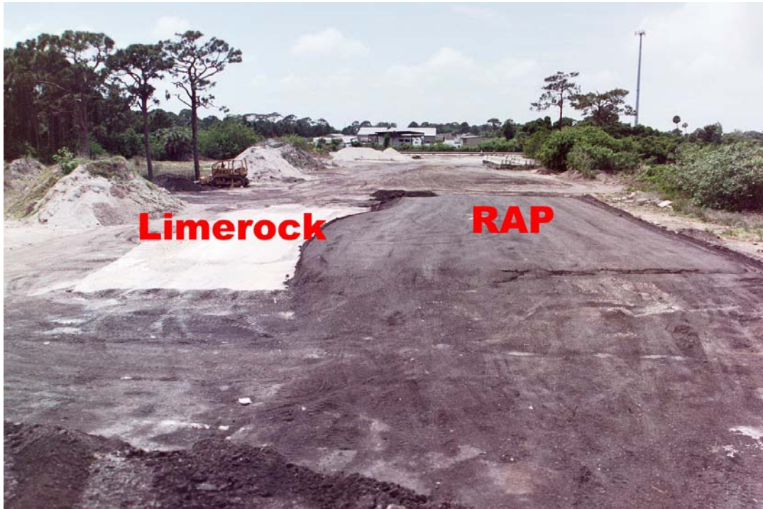
Figure 3.4 Completed Highway Materials Test Field Site
