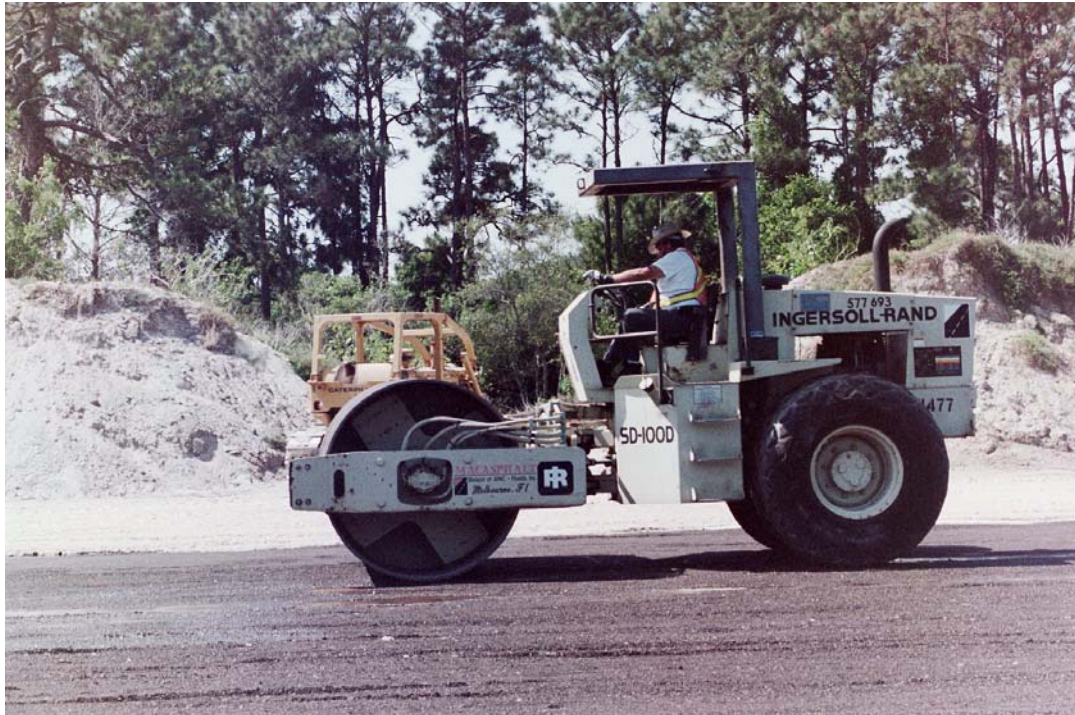
Figure 3.3 Vibratory Compaction of 1 st Lift
