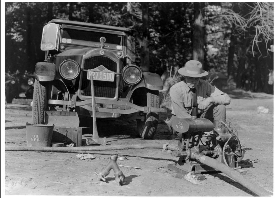
Figure 5: Portable fire pump, 1925. Courtesy, National Park Service, Yosemite National Park.
