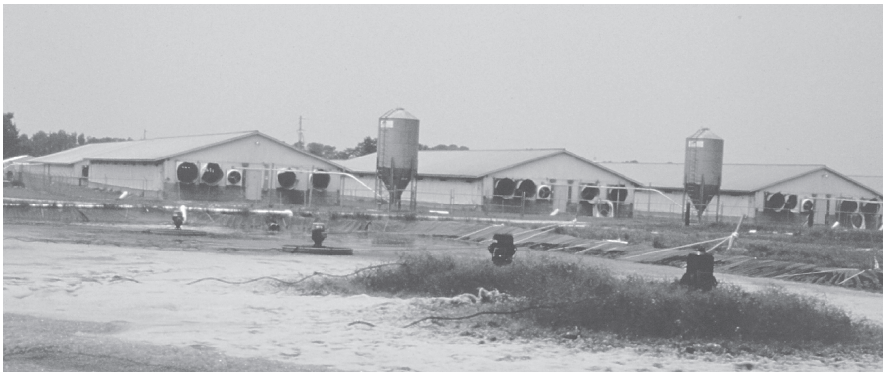
Figure 43-8. Aerated lagoons treating flushed swine manure.
