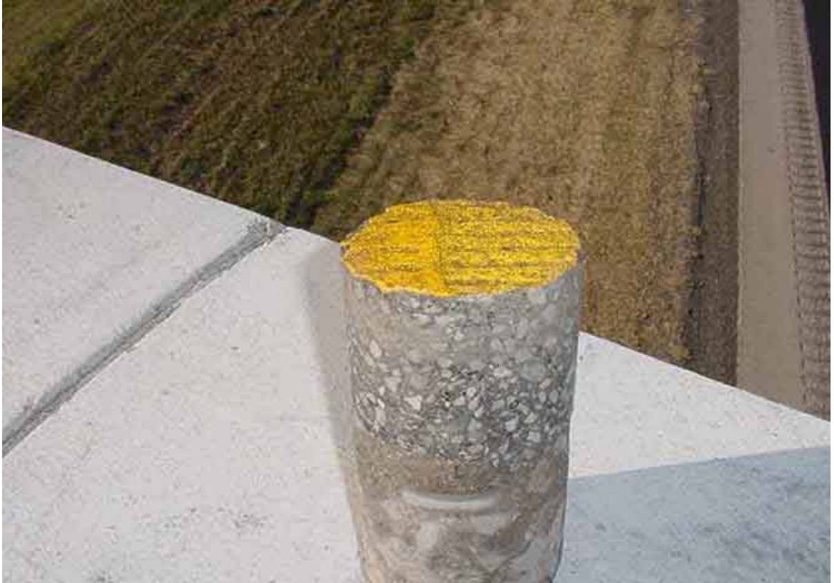
Core taken at centerline construction joint
