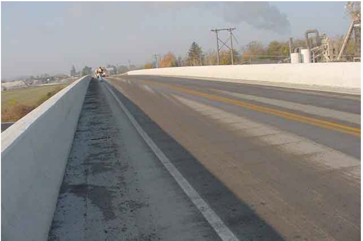
Wetting the deck prior to visual inspection
