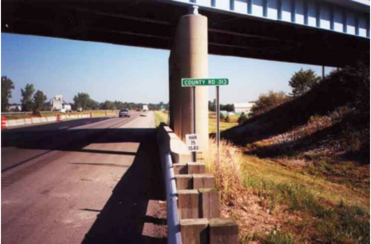
I-75 under bridge looking North
