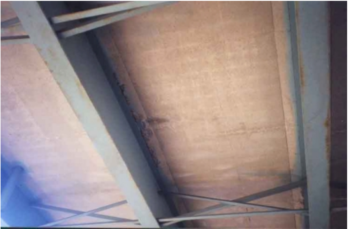
Minor leakage
