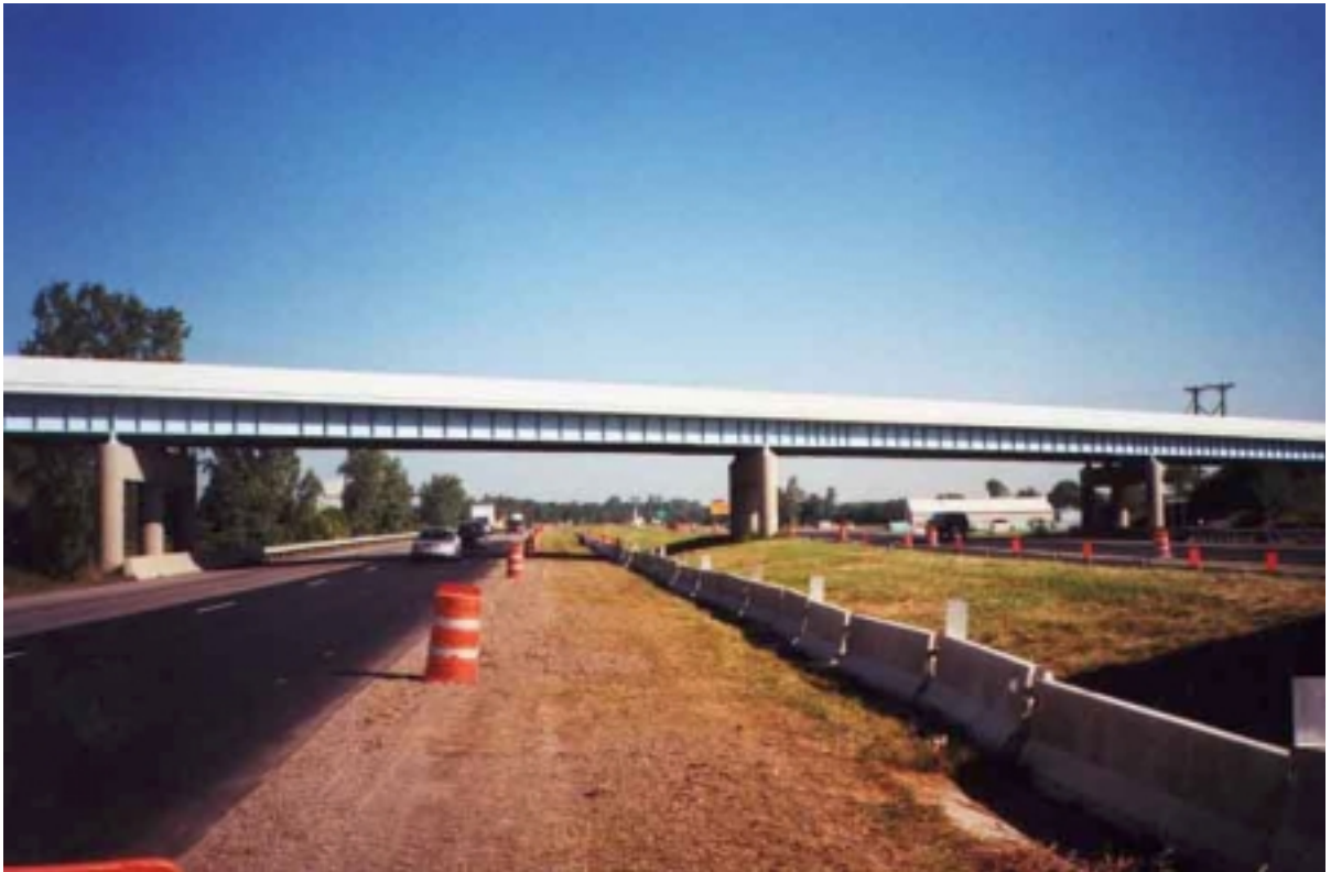
Looking at south side of bridge
