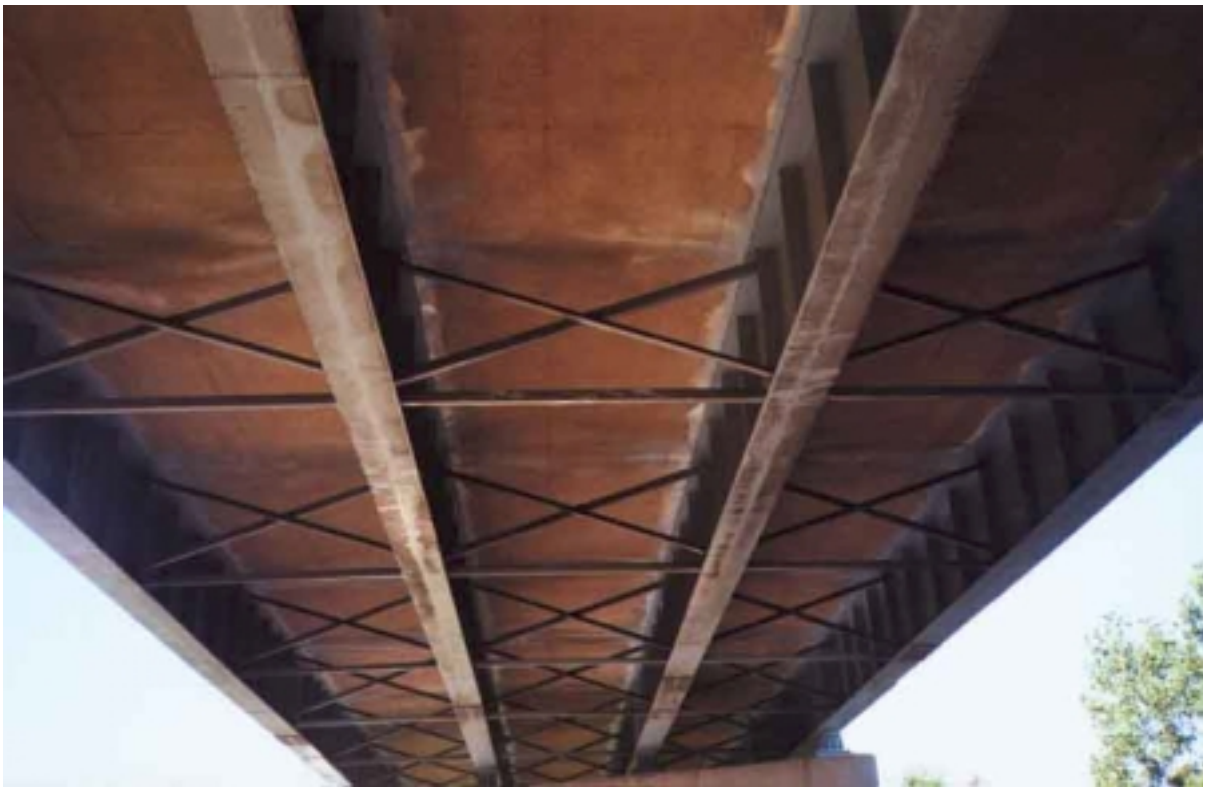
Underside of bridge looking southwest
