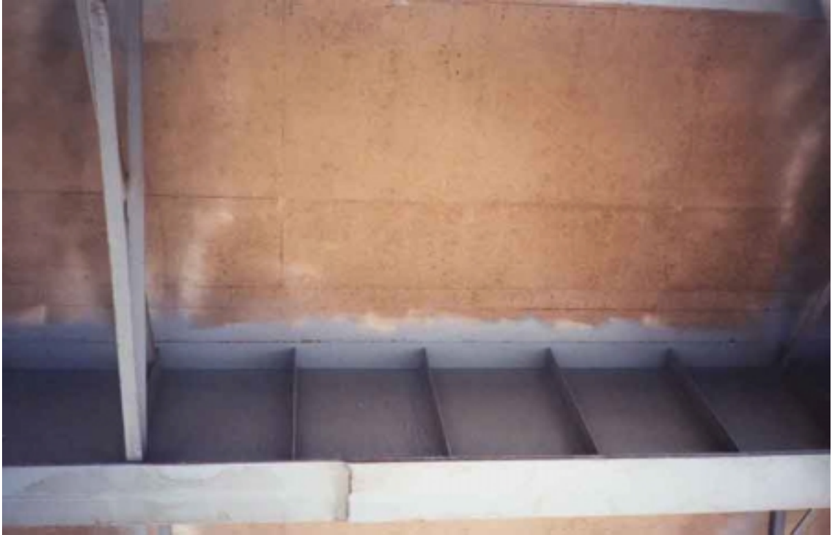
Typical underside condition
