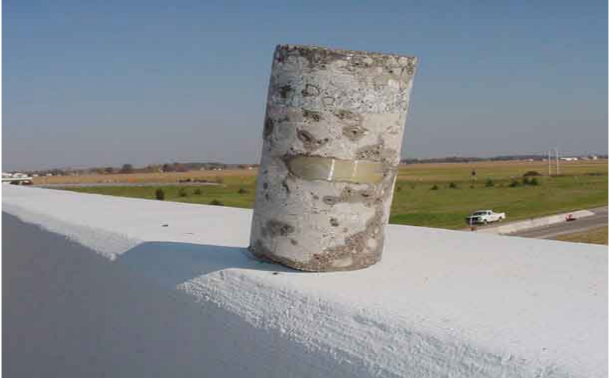
Core taken through the side of a reinforcing bar
