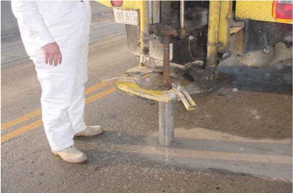
Drilling a core
