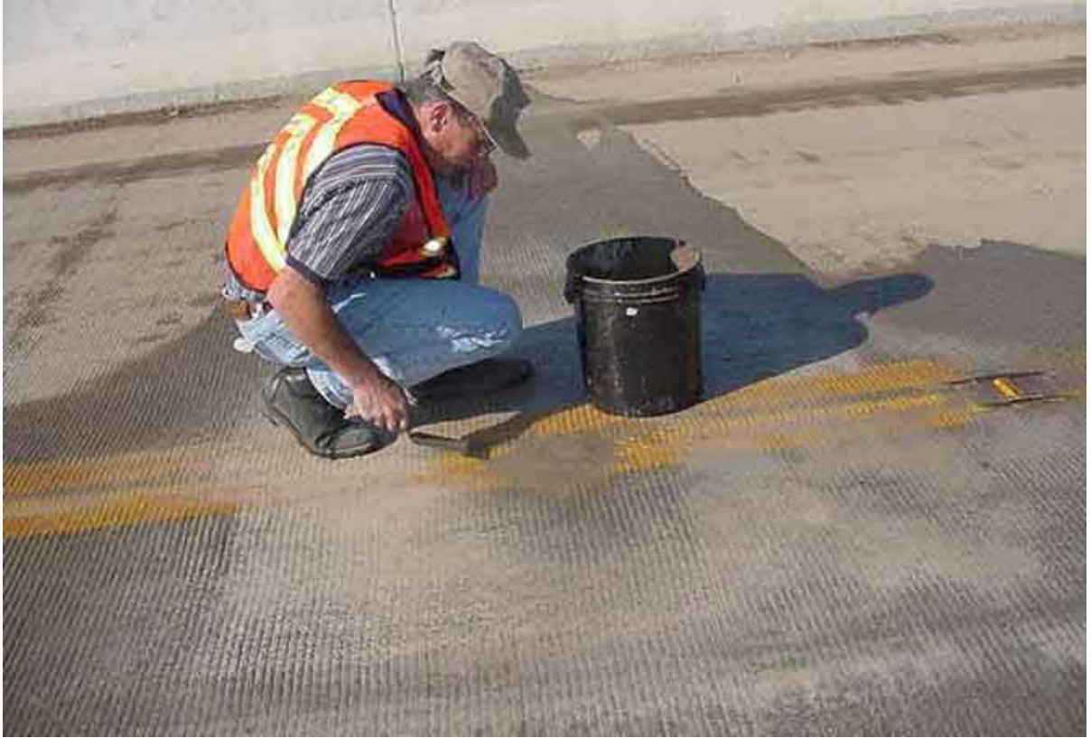
Patching core hole
