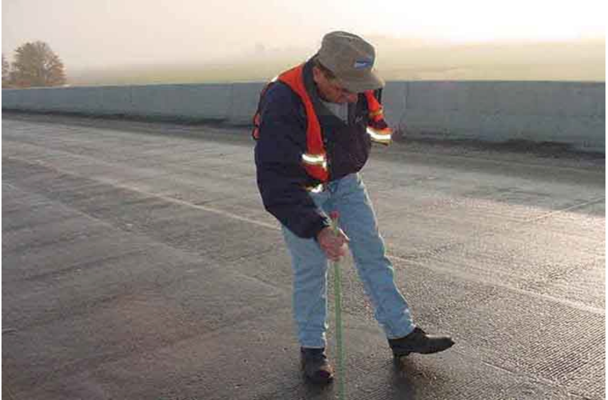
Sounding the deck
