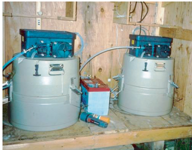
Figure 5.25 .Double monitor setup for sampling over a wide range of flow conditions.
