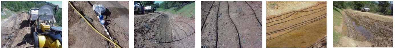
Acetic acid solution was metered in two sets of drip tape. Drip tapes were placed along the canal profile to insure complete coverage.
