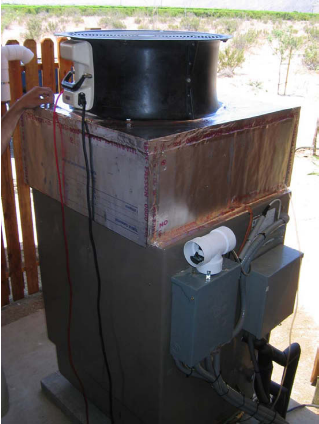
Figure 28. Fan-assisted flow hood installed on the Freus unit
