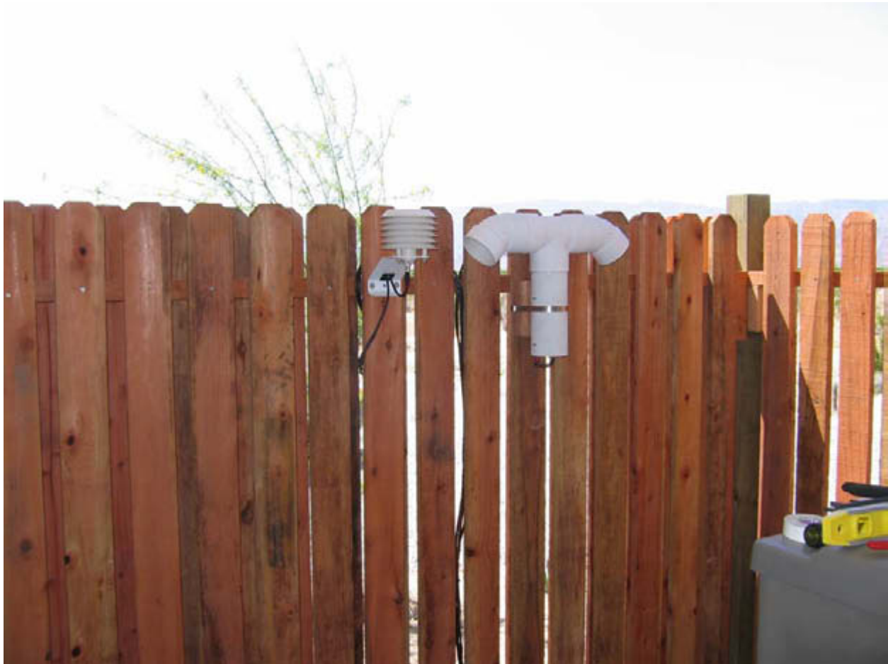
Figure 25. Vaisala temperature and RH sensors (left in plate shield) and custom forced-aspiration radiation shield with thermocouples (right, white PVC) installed at fence surrounding Freus condensing unit
