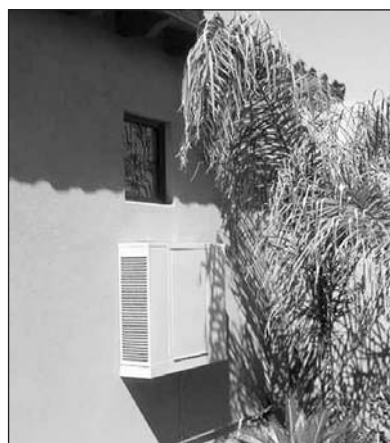
Figure 3. A new evaporative cooler by Adobe installs in the wall at the side of a home (photo and schematic).
