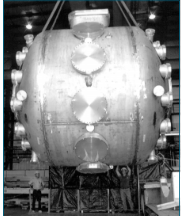
Construction of the National Spherical Torus Experiment (NSTX) progressed rapidly. The 23,000-pound vacuum vessel for NSTX arrived at the Laboratory on August 5, marking a major step in the construction of the new device. Earlier in the summer, the world's tallest ohmic-heating solenoid was delivered to PPPL and lowered over the inner toroidal field coils of NSTX, which were also major milestones in the assembly of the project.
