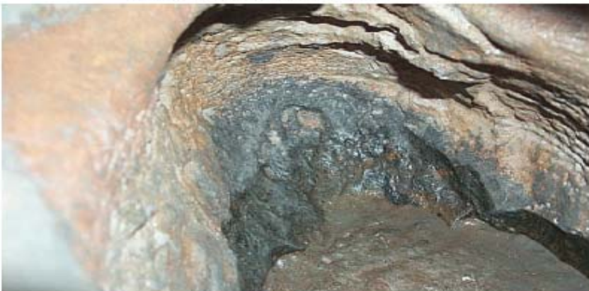
Close-Up View of Cavity
