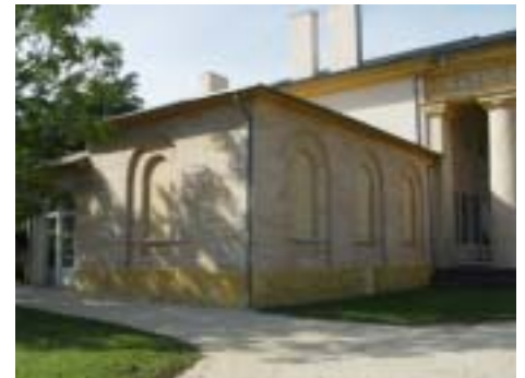
Arlington House: South Wing windows covered with plywood
