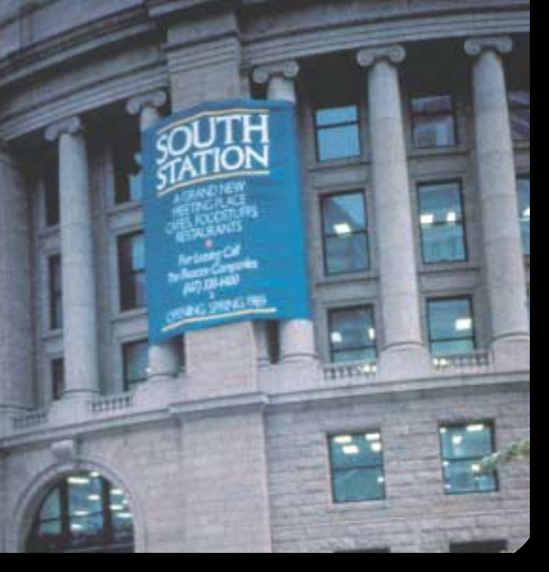
Boston South Station's façade during renovation.
