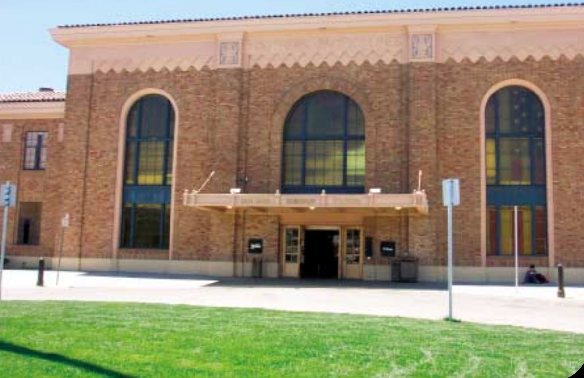
The Diridon Station, located in the renovated 1935 Southern Pacific train depot, is an anchor for redevelopment in San Jose.
