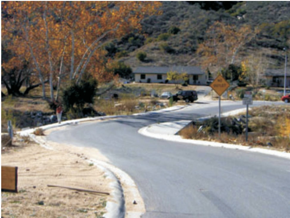
View of Sycamore Road crossing of Pala Creek, looking west (12/22/05)
