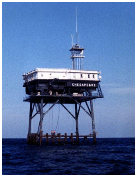
Figure 6. Chesapeake Light platform 25km off the coast of Virginia. CERES has developed and supported this as an ocean background BSRN and AERONET site.
