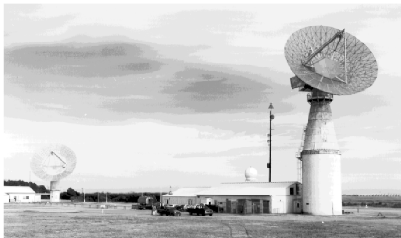
Figure 3-20. Atmospheric Sciences Research Facility
