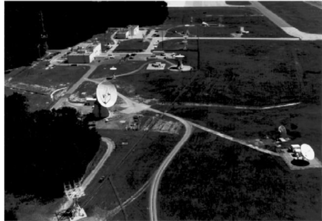
Figure 3-12. Range TM Facility and WOTS
