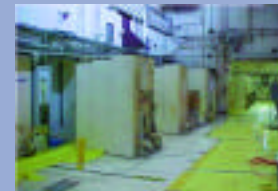
Seven Hot Cell doors were removed- each weighing over 20,000 pounds.
