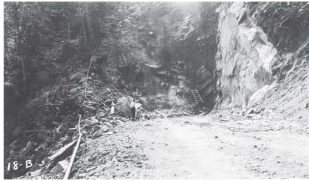
North End of Marys Rock: Although the road bed from Panorama to the north end of the proposed Marys Rock Tunnel had been temporarily graded by late Autumn 1931, the contractors would not break through from the south until January. Note the highly unstable rock slopes above what would become the tunnel portal. These slopes later required the construction of terraced retaining walls.
