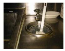
hour operating day, a dipper well will use 175,000 gallons a year and cost over \$1,000 in water and sewer charges. If the dipper well is flowing hot water, then you will pay another \$1,000 for the energy to heat that water. That's over \$2,000 a year for one little spigot!
